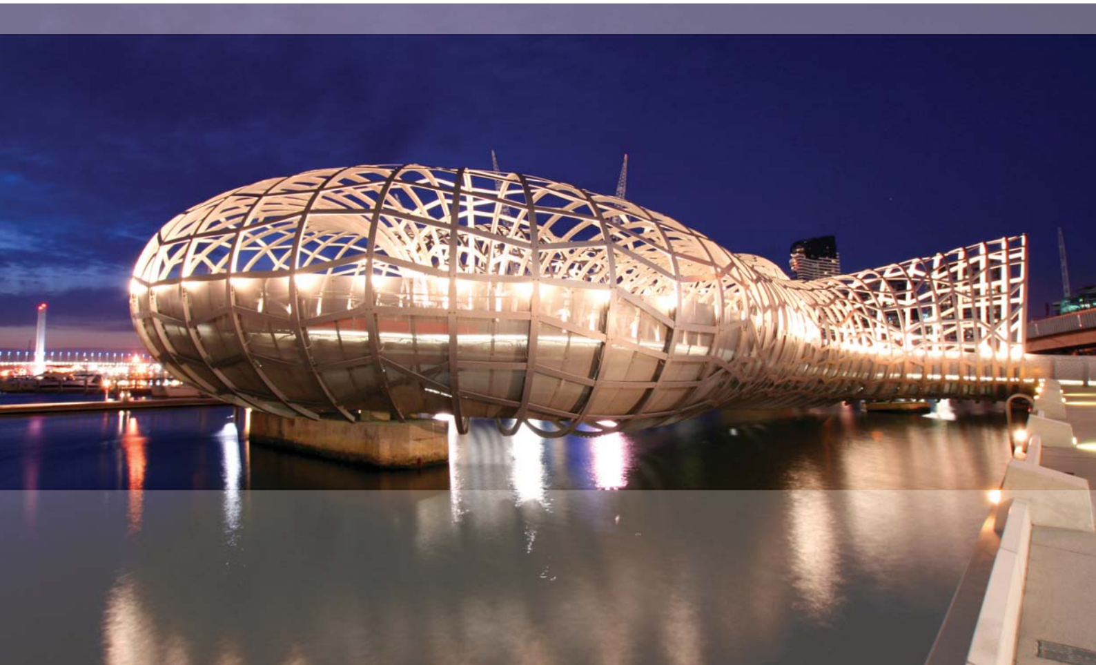
WEBB BRIDGE DOCKLANDS, MELBOURNE
