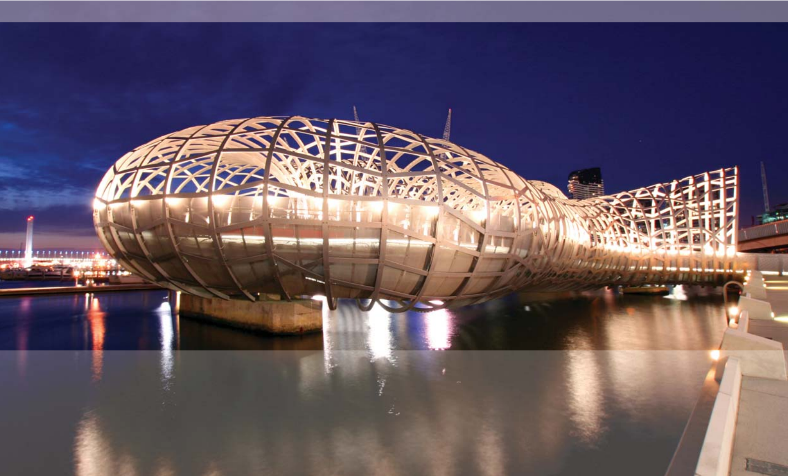
WEBB BRIDGE DOCKLANDS, MELBOURNE
